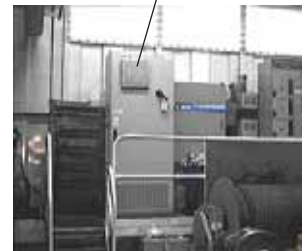
RC2000 Installation in Crane Machinery House
